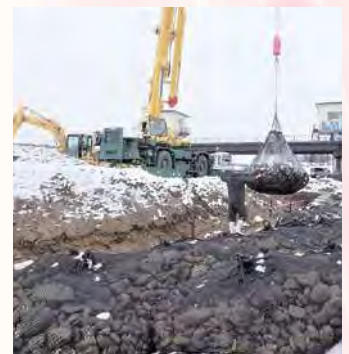
▲塩川頭首工護床補修
